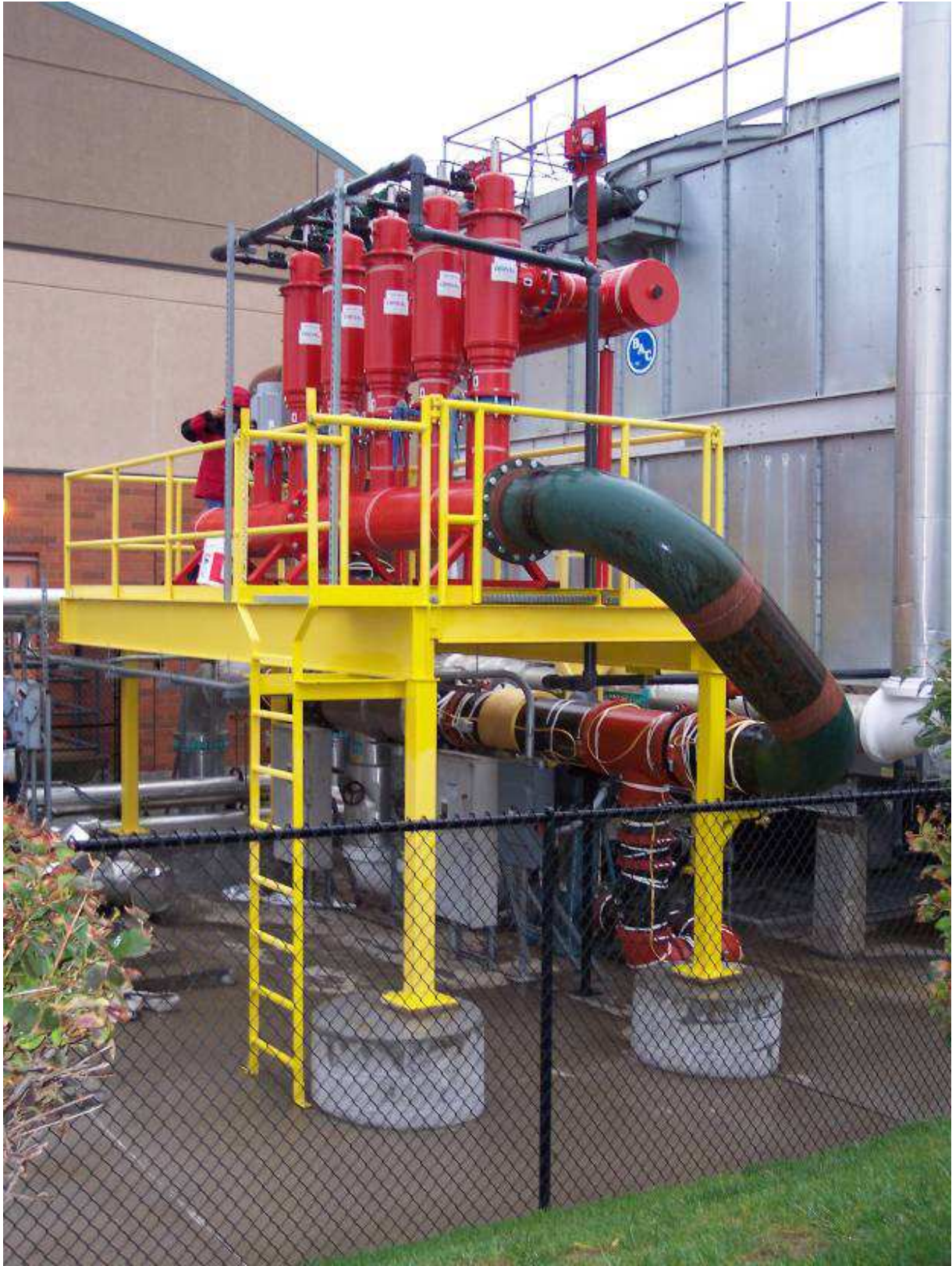
Figure 3. Filtration System Layout
