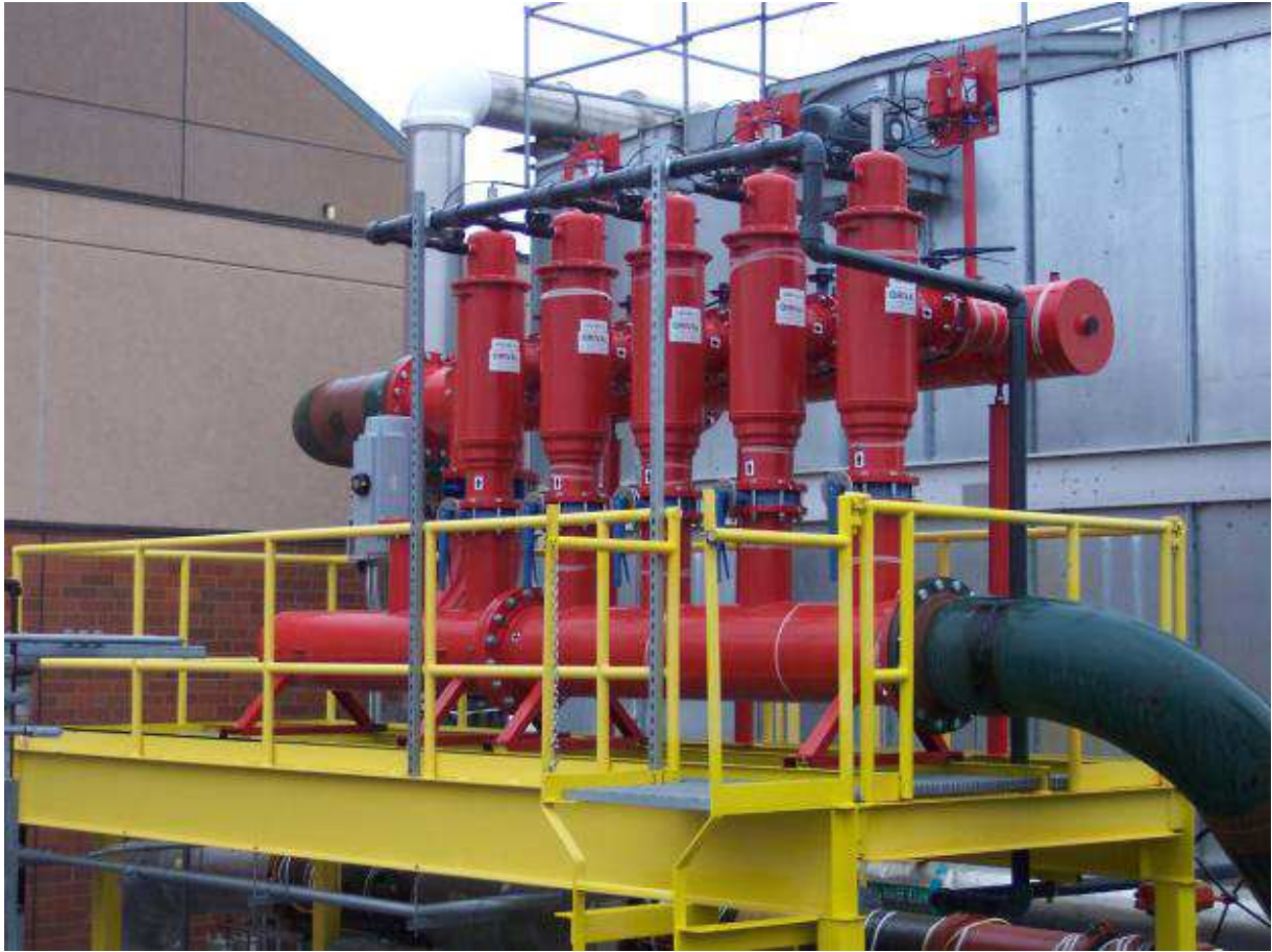
Figure 2. ORIVAL Five-Filter System
