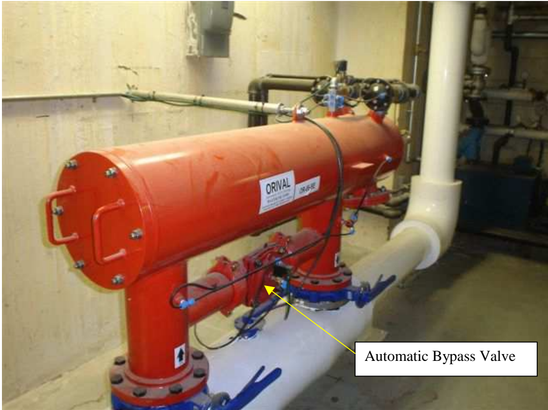
Figure 1. Filter Installation
