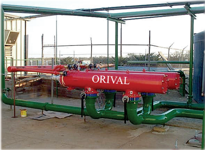
Two ORI-10-PE units filter reclaimed water for turf irrigation in central California
