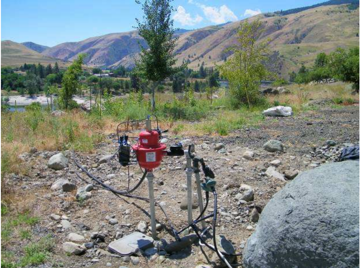
Picture 1. Filter Installation
